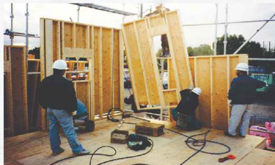
Assembling Nelson panelized walls in Japan
