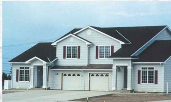
Duplex, Malmstrom Airbase
